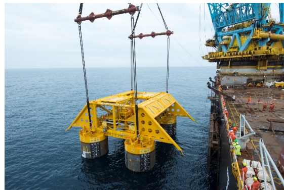
The installation of the compression modules on the Åsgard field – © Equinor
